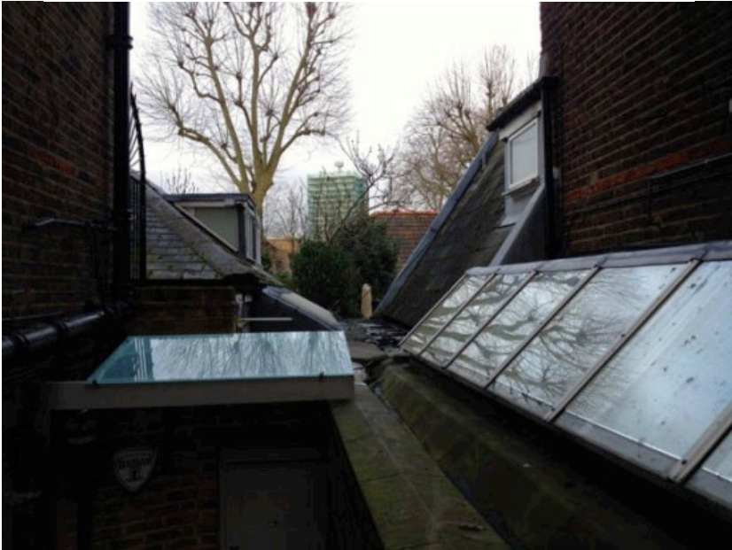
CLOSE UP VIEW OF GAP BETWEEN NOS. 76 & 74
