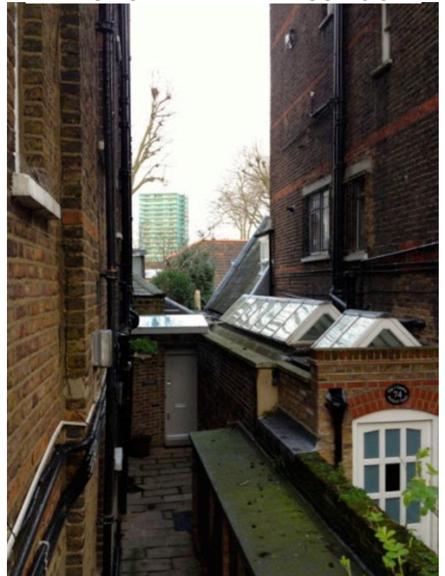
VIEW OF GAP BETWEEN NOS. 76 & 74
