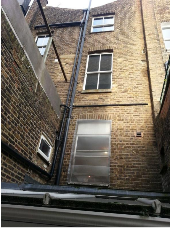
Rear elevation – Ground, 1 st and 2 nd floors
