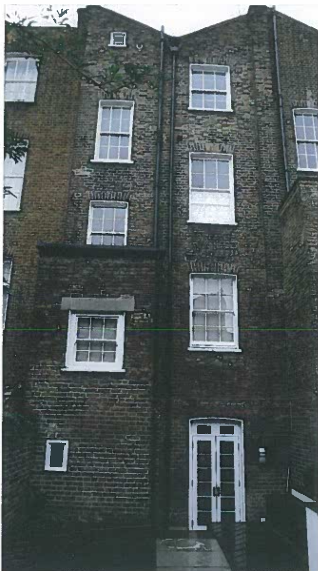
3. View of rear facade showing sash window nos: W7 W8 W9 W10 W11 W12 and door D1 changed from single to double glazing (see drawings 1, 2 and 3)
