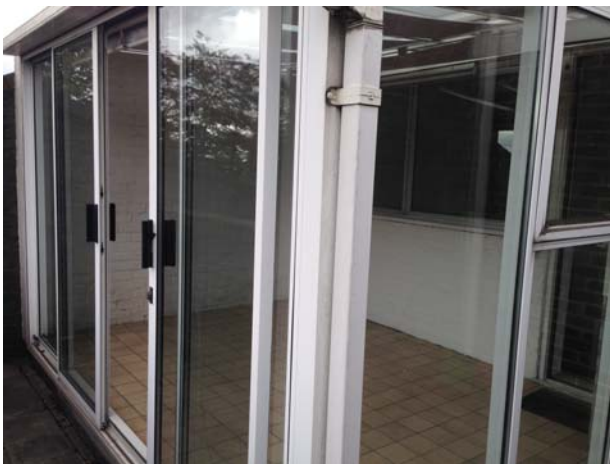
View to the conservatory of 1D at roof terrace level
