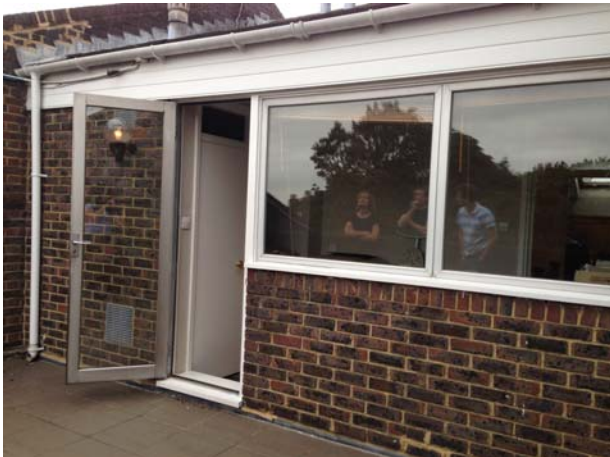
View to the rear elevation of 1C at roof terrace level
