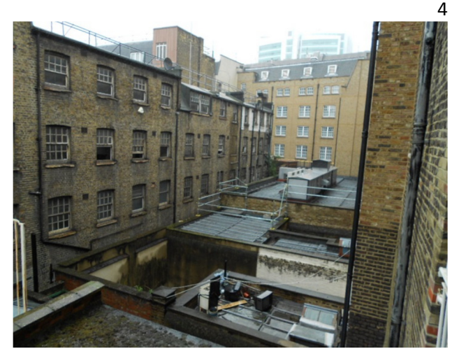
View of Suffolk House from rear of 64 Grafton Way
