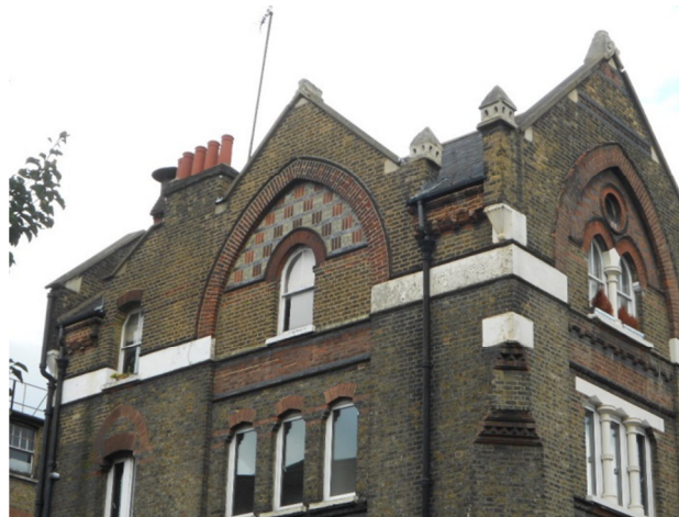
Gothic arches and unusual eclectic masonry detailing
