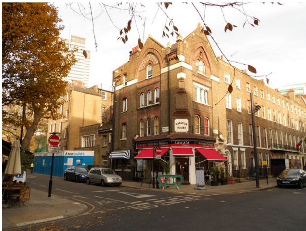
Existing view from south
