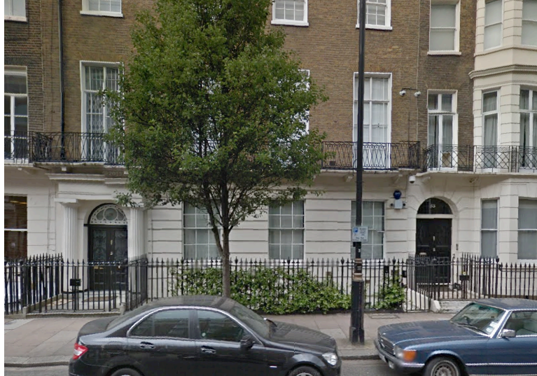
Figure 6: Gates and railings along Great Cumberland Street
