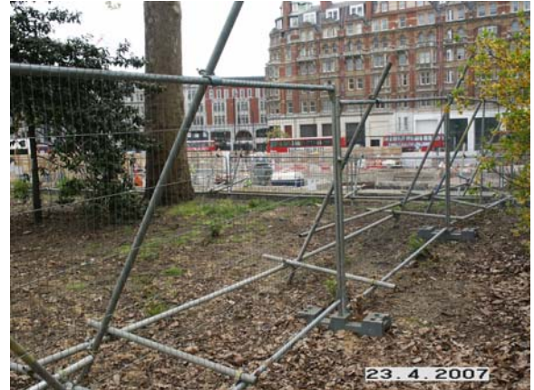
Effective fencing in position
