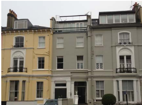
PHOTOGRAPH 11 : Context (No.44 Regents Pk Rd) - Example of non-subservient additions, that detract from the original building form
