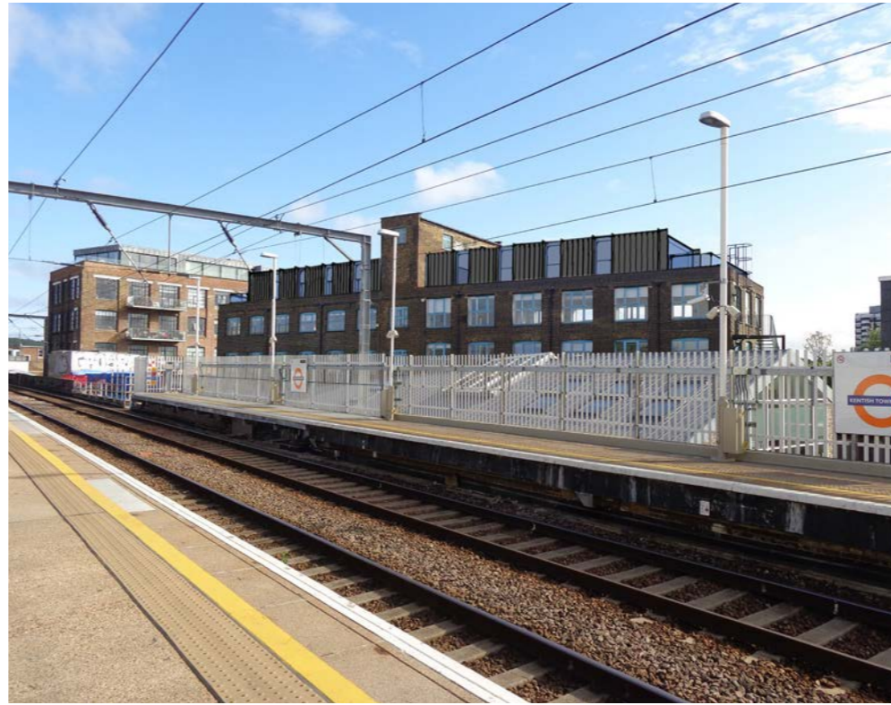
View from Kentish Town West Overground Platform Proposed _ lightweight roof extension; facade echoes rhythm of existing building
