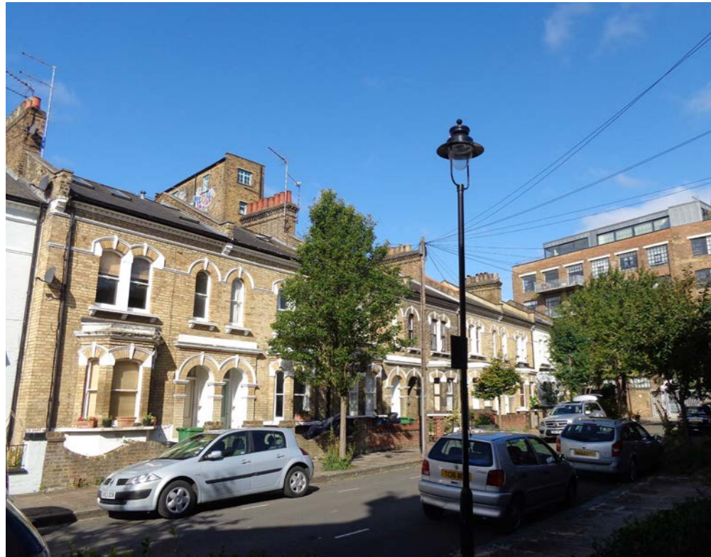
View West across Ryland Road Existing _ showing two storey core overrun
