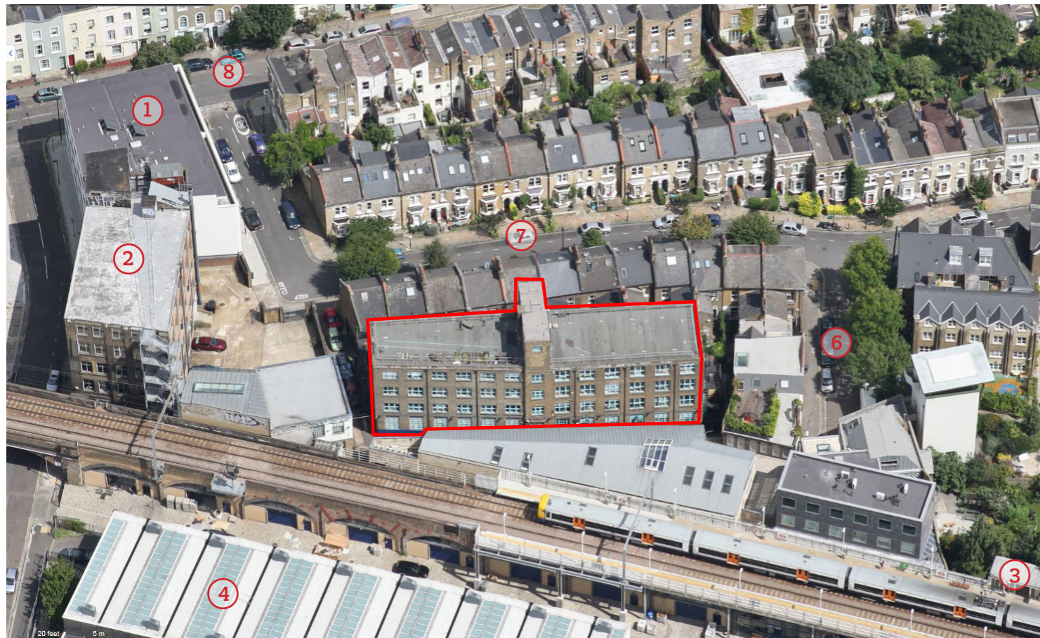
Aerial view of West elevation
