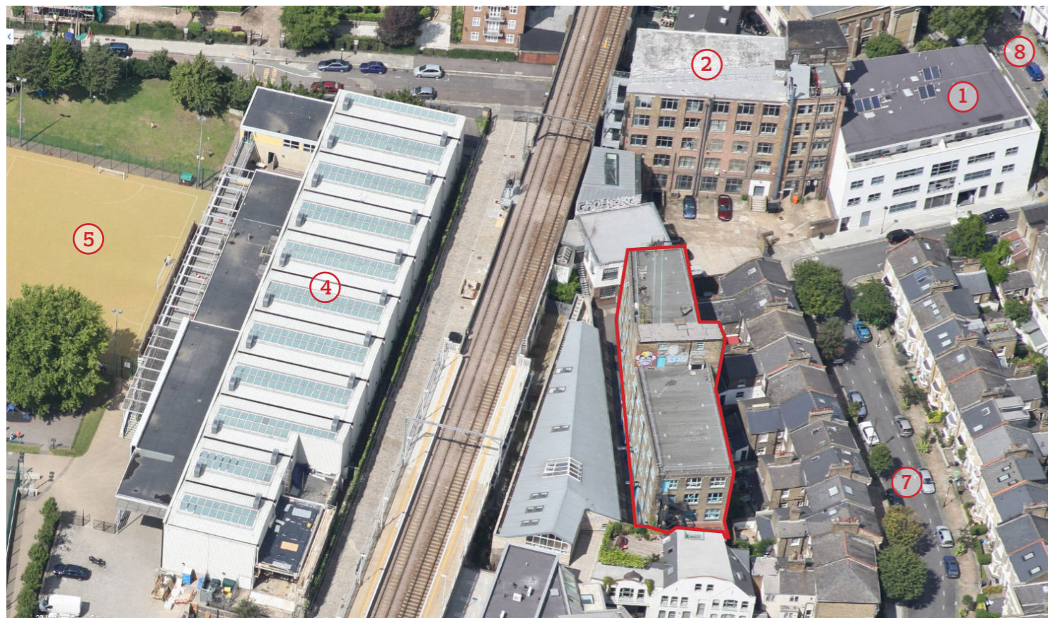
Aerial view of the South elevation
