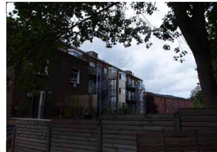
Neighbouring buildings from the back garden of the site
