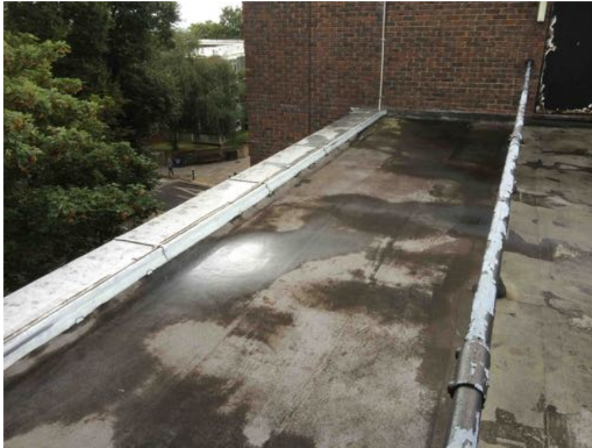
Roof of existing building
