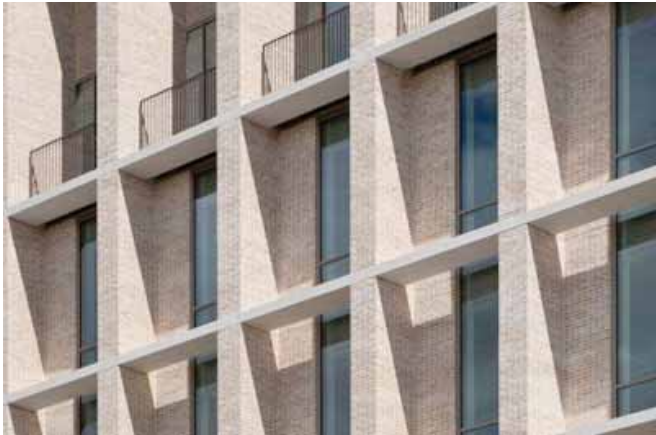
The material selected for Block C is a machine made clay stock brick with a light variegated texture, with flush matching mortar
