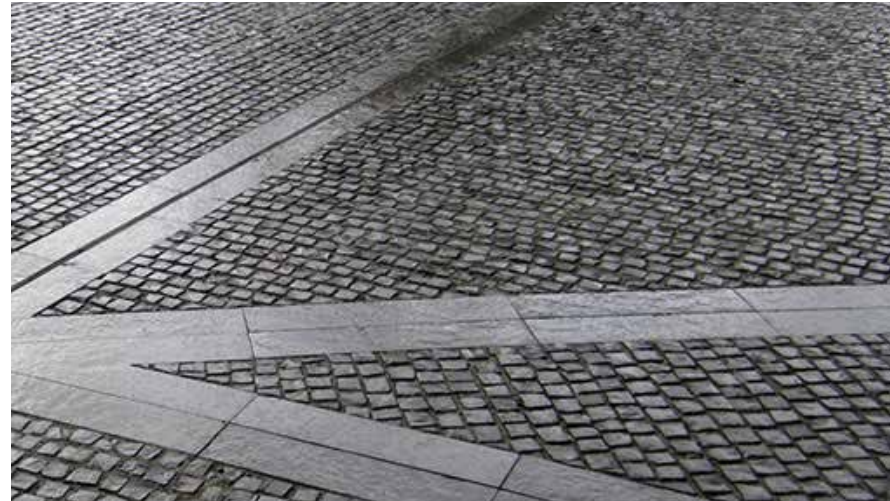
Feature granite sett paving and banding to parking and service bays
