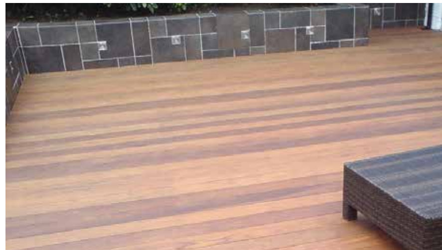
Timber decking to roof level
