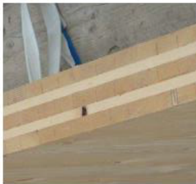
A cross laminated timber panel formed of 5 timber boards
