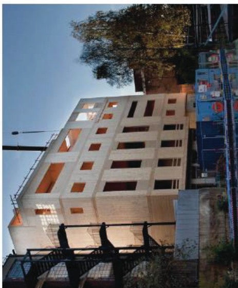
Cross laminated timber shell finished
