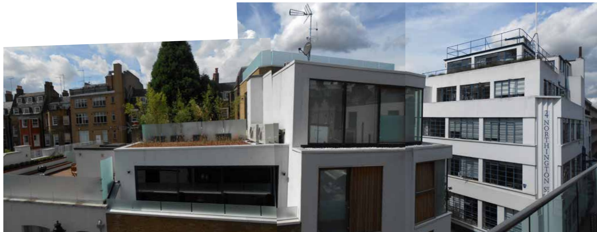
Roof Terraces on Opposite Side of Street
