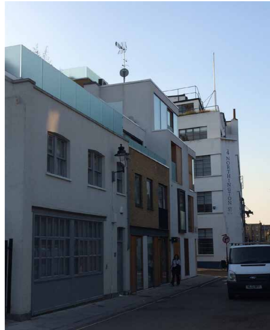
Existing Roof Terraces on Opposite Side of Street
