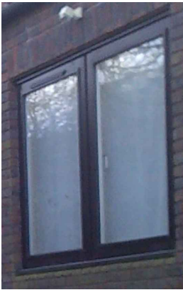
New wood window double glazed plain windows to match exiting
