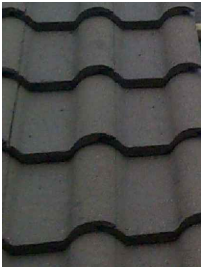
New single shire concrete roof slates to match existing
