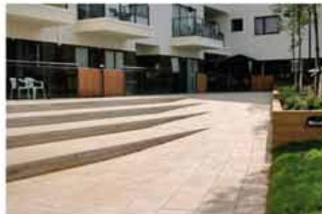
EXAMPLE OF RAMPED ACCESS WITH STEPS
