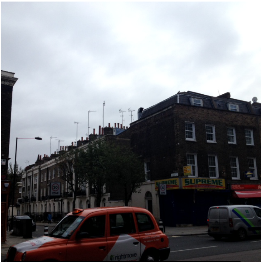
View of Nos.290 - 292 Gray's Inn Rd and Frederick Street
