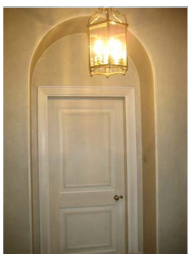
4 | PHOTOGRAPH TYPICAL EXISTING DOOR 30 | NTS
