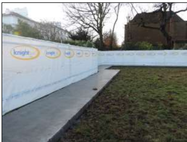
Photo 1: Concrete slab ground protection with heras panels on a scaffolding frame at the rear. Southern corner of the site.
