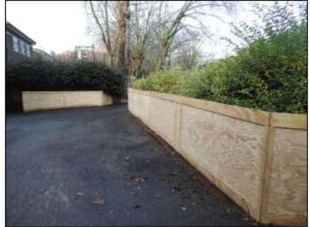
Photo 4: Low plywood panels used for protecting the root protection areas at the front of the site.
