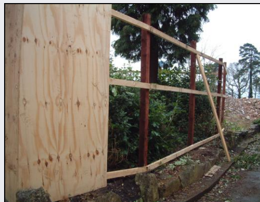
Board specification on secure wooden posts
