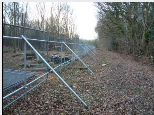
Heras fencing wired to scaffold braced posts
