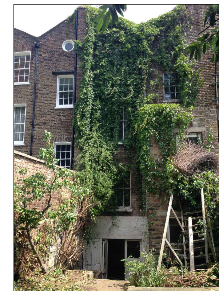
Photo Showing Existing Rear Elevation
