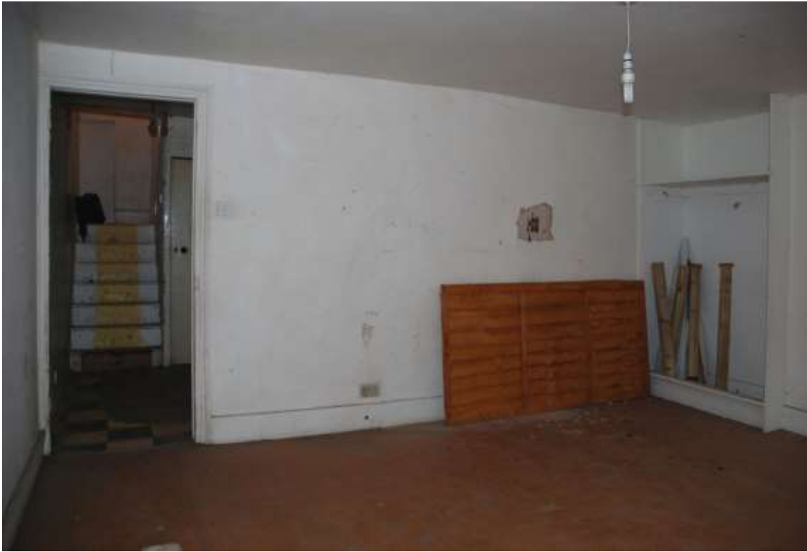
Fig.30: The internal dividing wall, from the front of the basement
