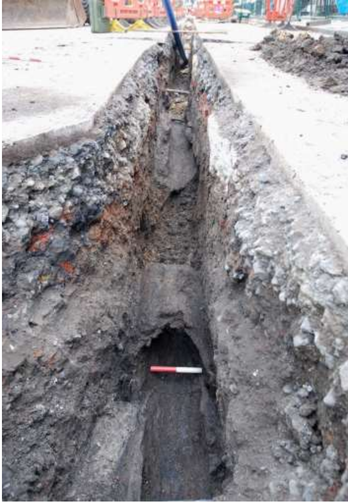
Fig.15: View of the exposed timber piping, looking south (0.2m scale)
