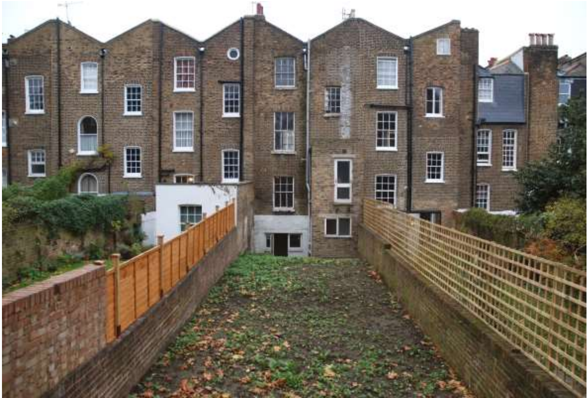
Fig.24: A general view of the rear of the property
