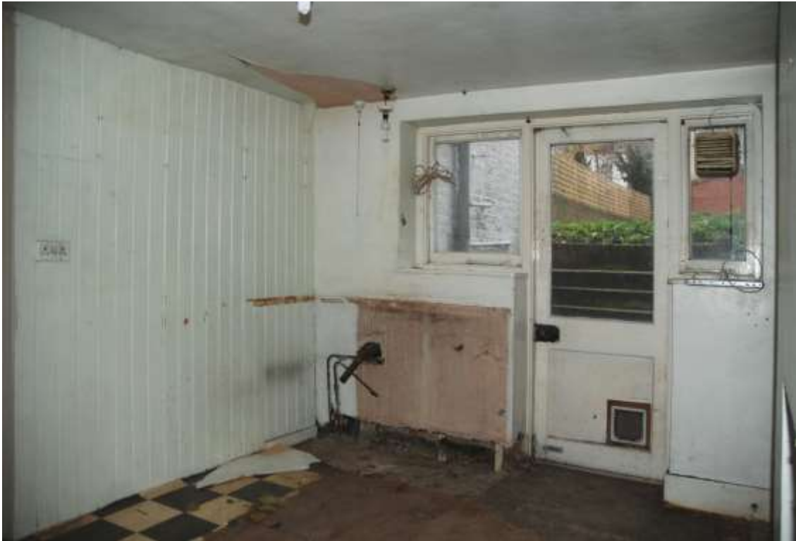
Fig.32: The rear of the basement, looking out into the garden. The door and windows are fairly recent, and to judge by the latter may well have been altered in size/position
