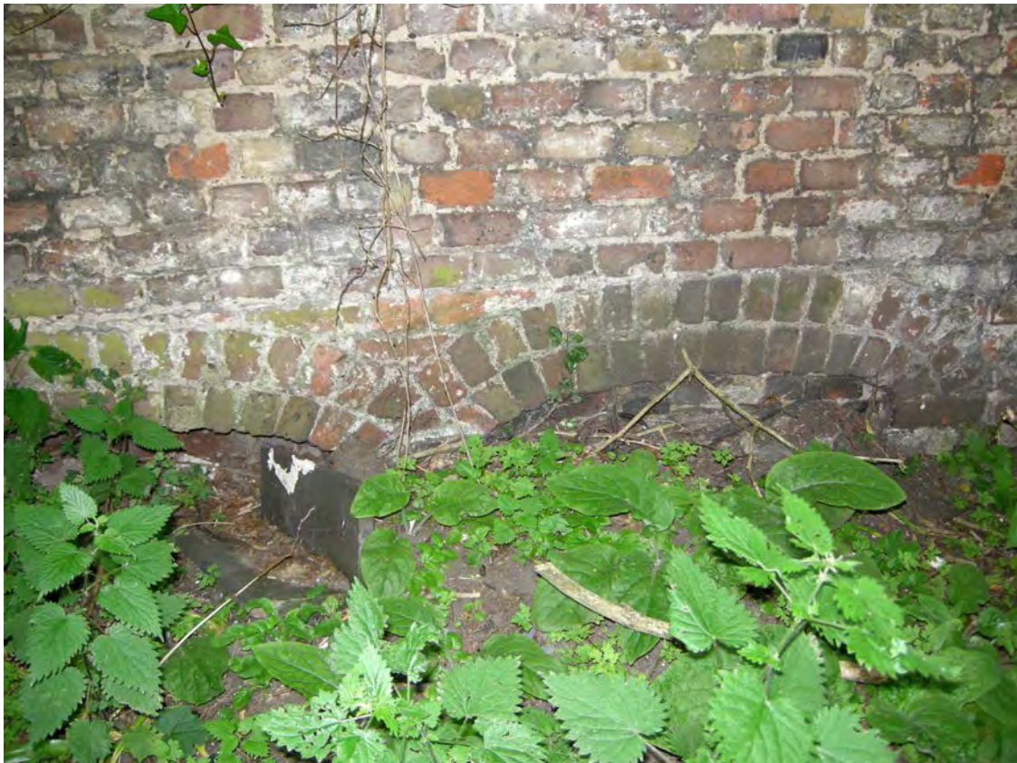
Fig 16 Bottom of north-east wall of store along south-west wall of 6 Streatley Place; view looking south-west (MOLA Photo 16.06.2014)
