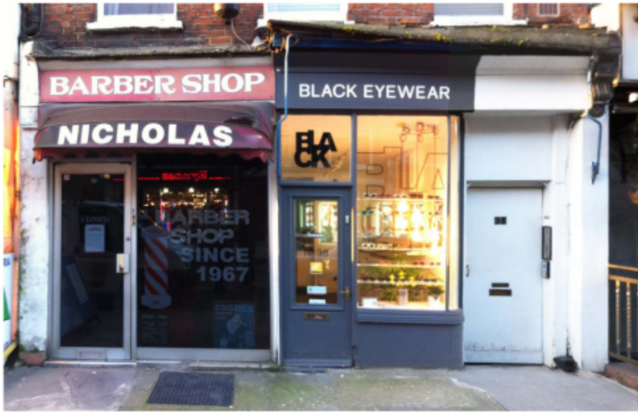
Shopfronts on site today
