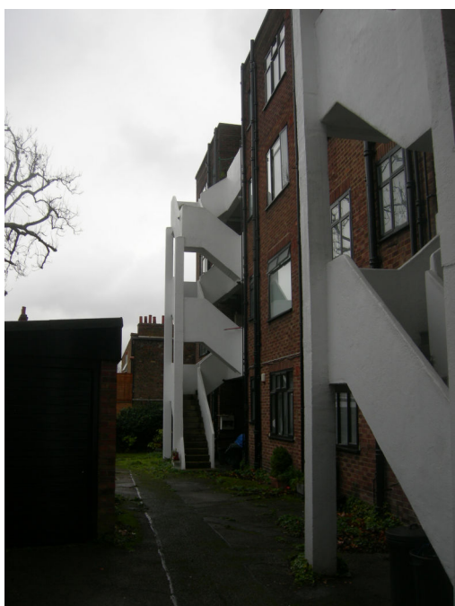
5 Rear - view south
