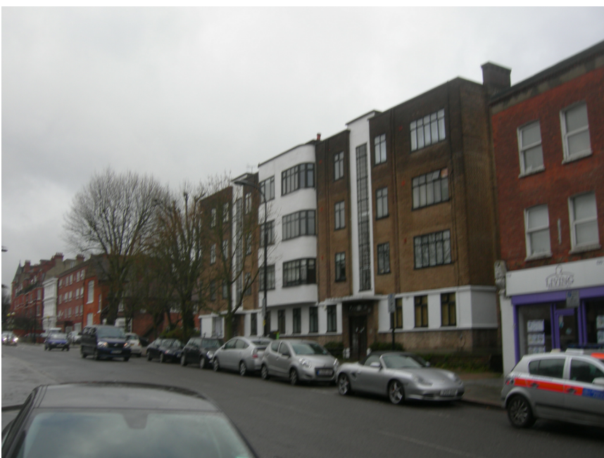
2. Fortune Green Road - view north
