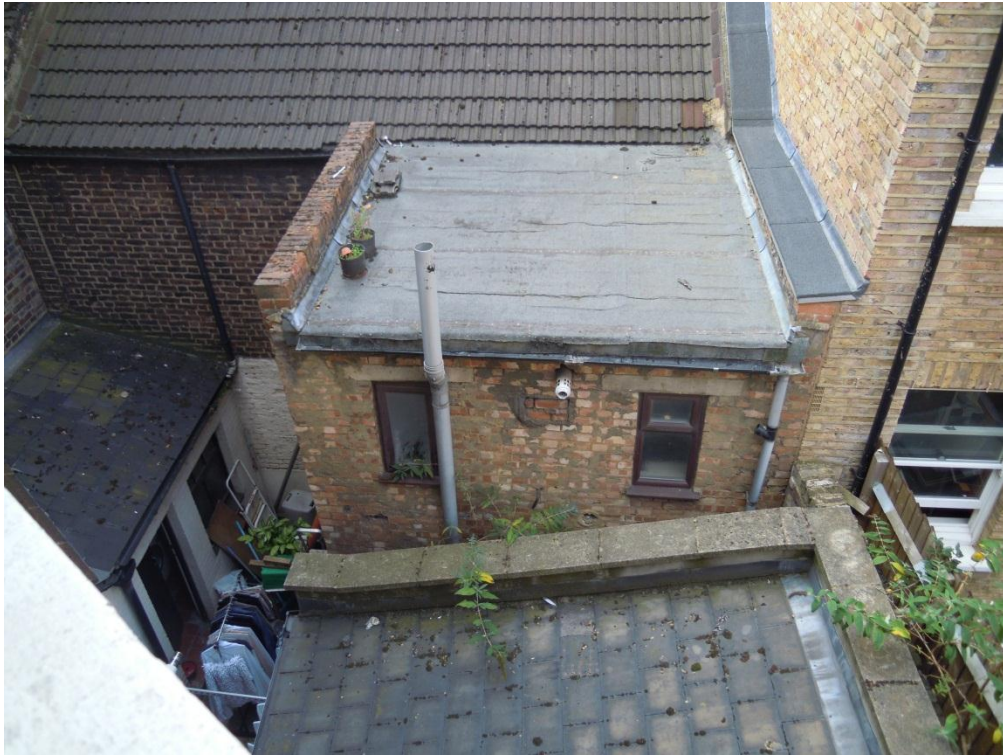
Rear wing of application site
