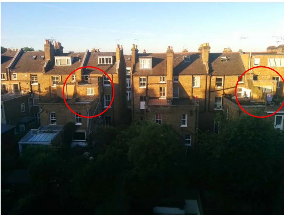
Example of other 2 nd floor extensions in immediate surroundings (Sherlock Road).
