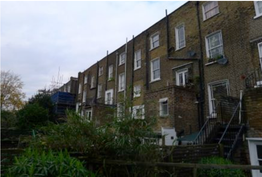
REAR ELEVATION LOOKING WEST, PAST NO.140
