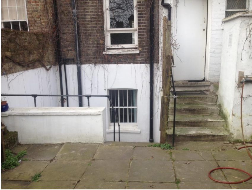
Photo 04 – 106 Albert Street–Rear elevation showing basement and ground floor levels.
