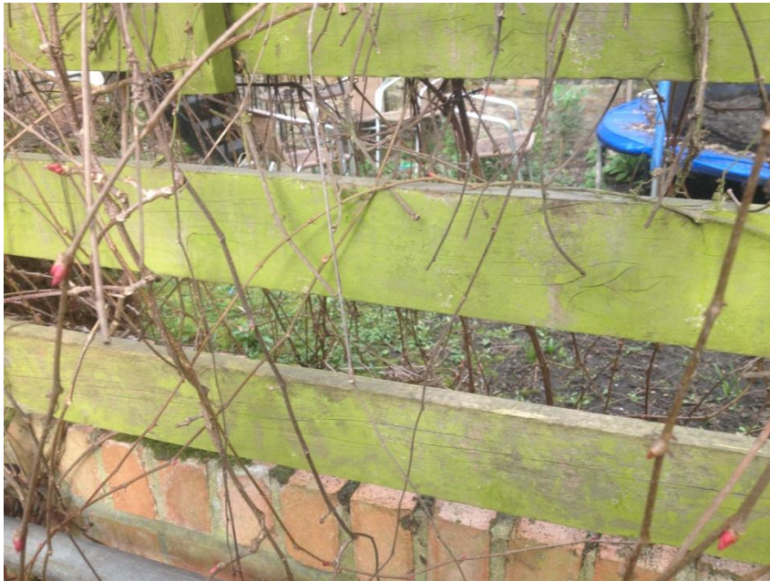
Photo 01 –108 Albert Street–Garden level approximately similar to 106 Albert Street garden level.
