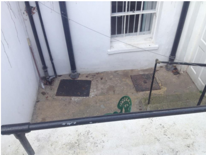
Photo 05 – 106 Albert Street–Existing basement level showing drainage.
