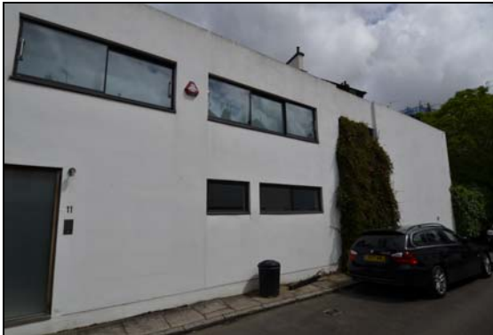
Figure 1. Main House (South Elevation)
