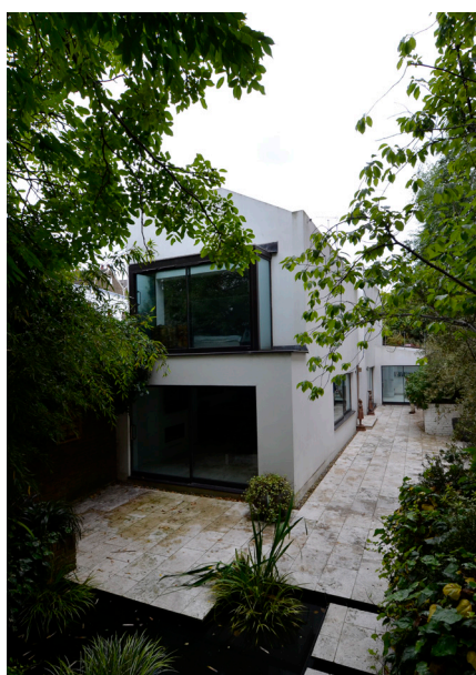
Photograph of the existing East and North elevations of the house from the garden gate.
