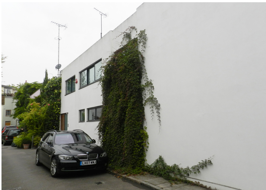
Photograph of the existing South elevation of the house from Albert Terrace Mews.
