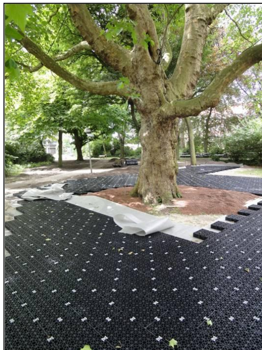
Figure 1. - Installed 'Arbraft' system around retained existing trees.
