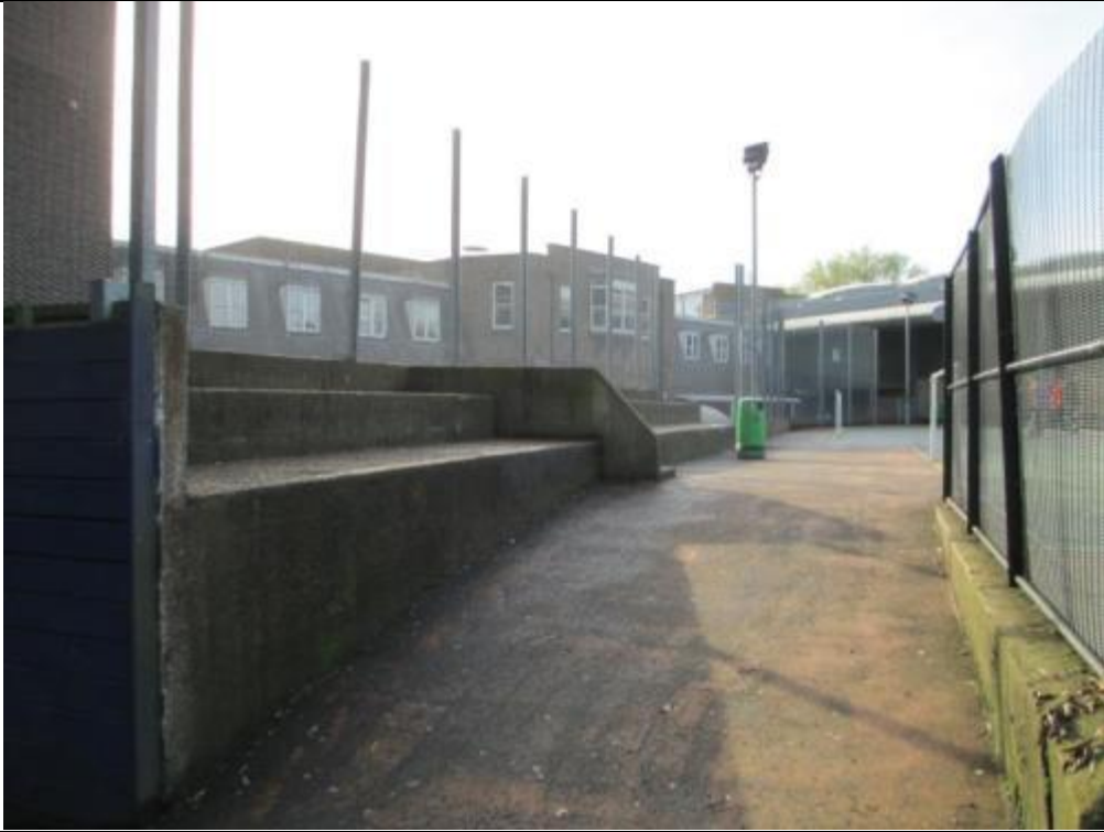
Rear of main building an Gym building with curved metal sheet roof
