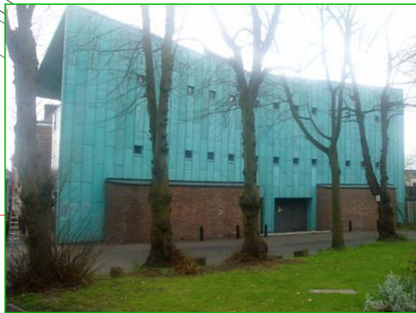
PHOTO 68: VIEW OF SOUTHERN ELEVATION
