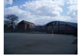
45. View of sports hall and school
