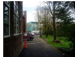
64. View to south elevation
