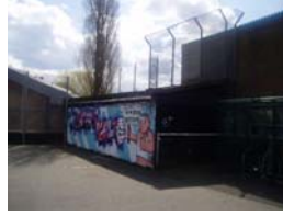
43. view of shed to western perimeter
