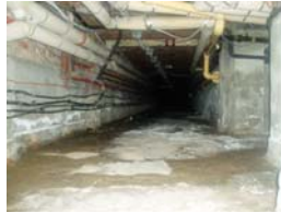
13. Void within boiler house
