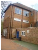
55. View of school building to eastern elevation
