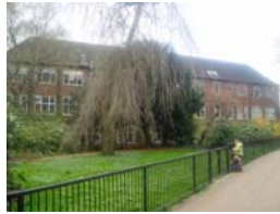
2. View of school from eastern boundary
