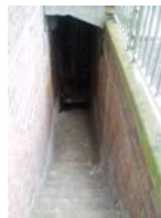
57. Stairs to boiler house
