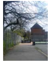
50. View of entrance road to eastern elevation
