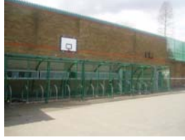
42. Bie shed to western perimeter
