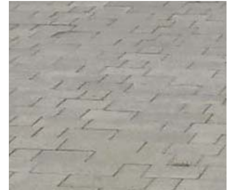
Concrete sett paving e.g. Andover washed by Charcon Colour: Silver Grey Sizes: 200x100x80mm
