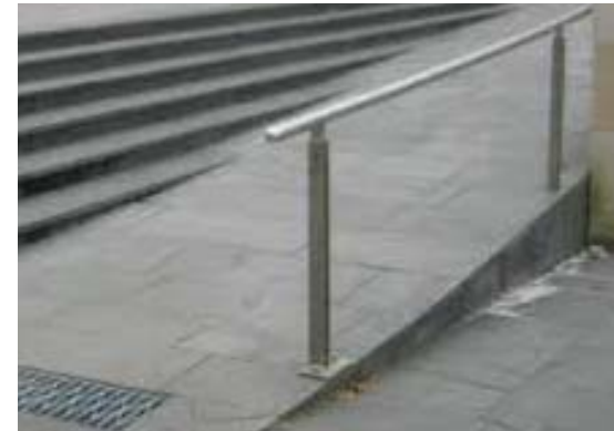
Stainless Steel Handrails to ramps
