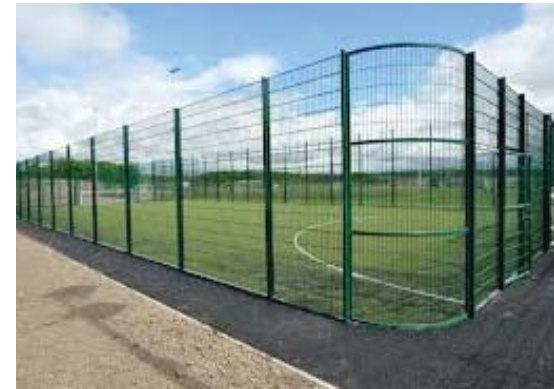
3 m weldmesh fence to games courts
