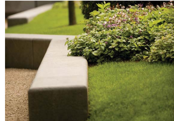
Cast-concrete retaining walls/informal perch/seat with exposed aggregate
