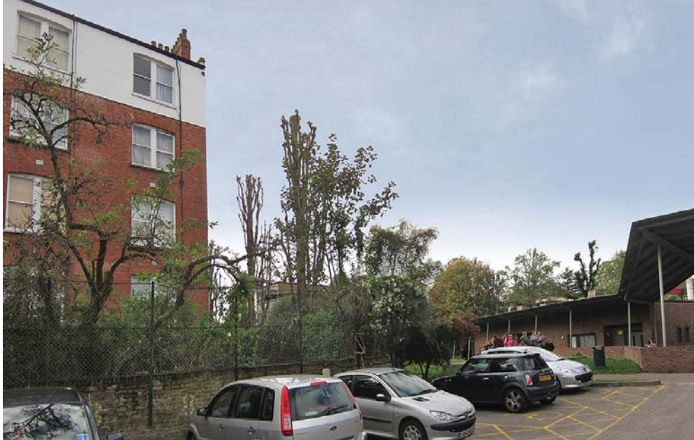
Existing view looking west along Lissenden Gardens
