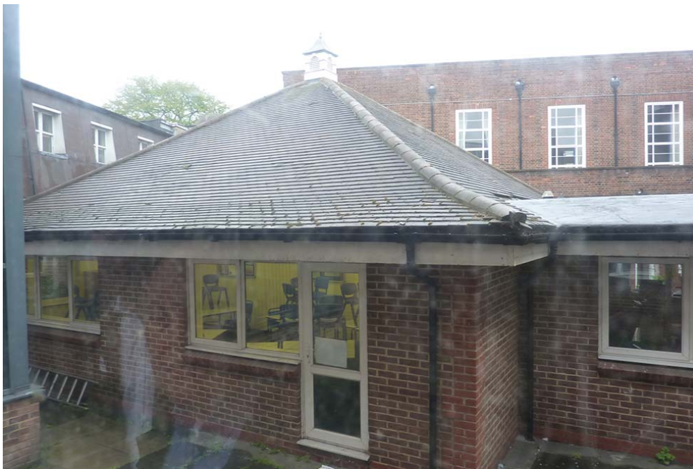
Existing view of the western central courtyard
