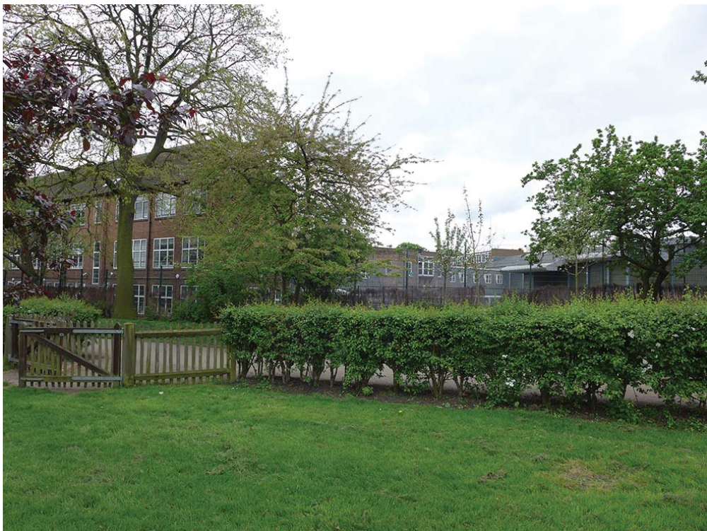
Existing view looking south-west from Hampstead Heath towards WES
