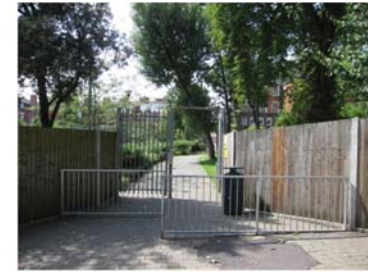
Pedestrian Main Entrance
