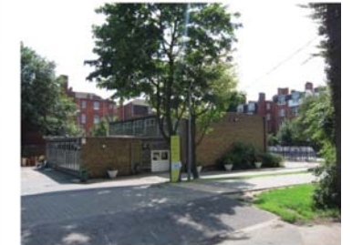
Existing Gym Building (Block B)
