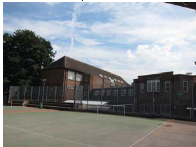
Looking over the MUGA to the rear elevation
