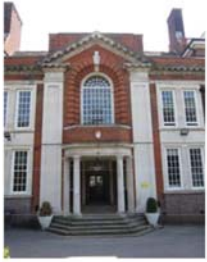
Main Entrance- Morant Building (Block E)
