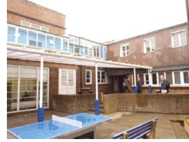
East Courtyard- towards dining entrance
