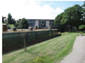
Courtyard Building and the Heath Building
