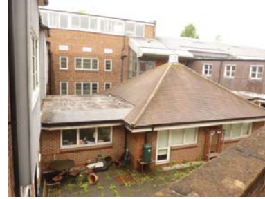
West Courtyard- view of MFL block
