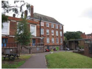
Rear view of the Morant Building
