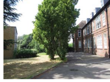
Front Façade looking towards PHS Heath bldg
