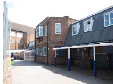
Rear view looking towards the kitchen
