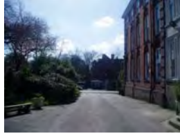
41. View to southern elevation
