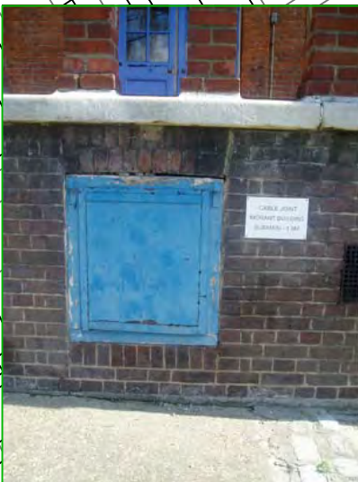
PHOTO 91: STEEL DOOR TO BASEMENT
