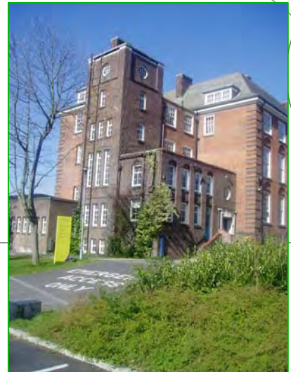
PHOTO 27: VIEW OF POTENTIAL LIFT SHAFT
