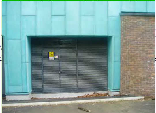
PHOTO 120: ELECTRICAL SUB STATION
