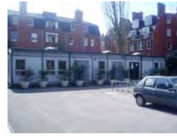
3. View of portakabins (site hut)
