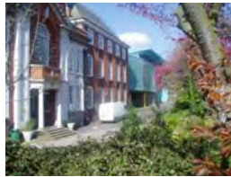
57. View to the north
