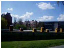
96. View of verrainders roof
