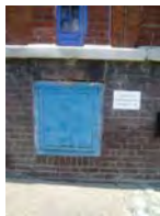
91. Steel door to basement
