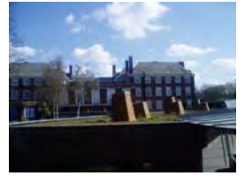
74. View of verrainders roof
