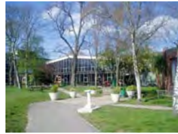
88. View of main hall
