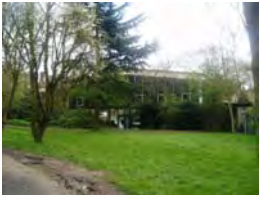
105. Main hall from the north
