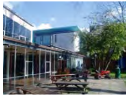
82. View of main hall
