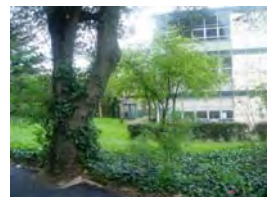
104. View looking from the north
