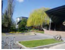
37. General view towards western elevation
