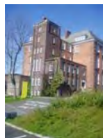
27. View of potential lift shaft
