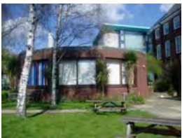
90. View of semi hexagon building
