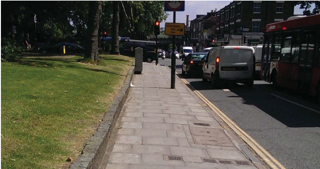
Photo 1 – Western Side Footway, Highgate Road (Southbound)
