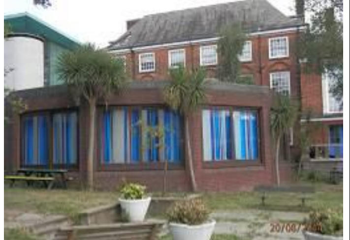
New brick addition at eastern end of block to be demolished
