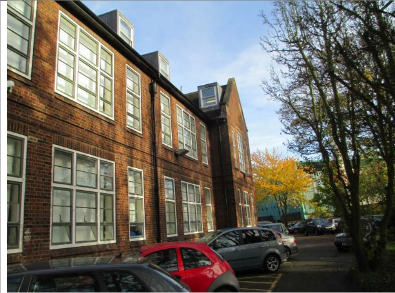
Plate 1: Frontage of main building (Trees are within the land controlled by the adjoining school)
