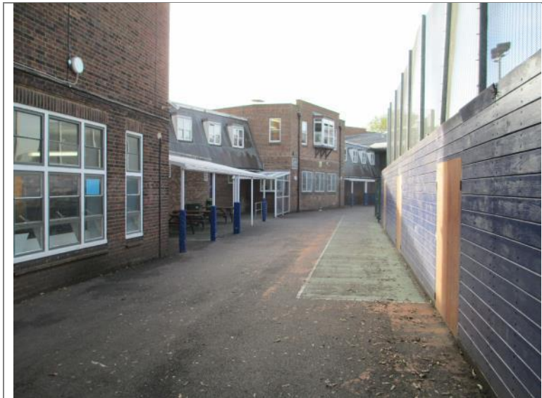
Plate 3: Rear additions to the main school building
