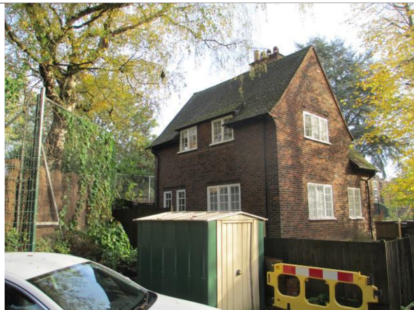
Plate 7: Residential property on the site
