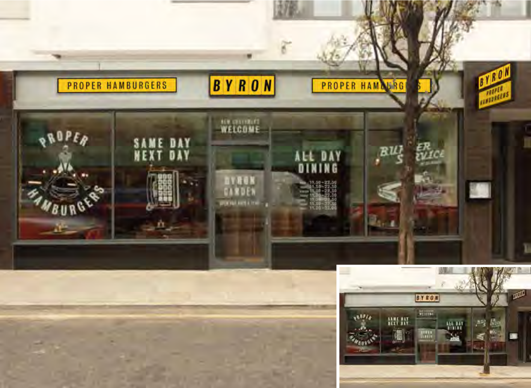
Proposed: Existing Byron lightbox to receive new panel finished Dulux 45YY 62/805 gloss. Existing Byron/ Proper Hamburgers projection sign to receive new panels finished Dulux 45YY 62/805. 2no new Proper Hamburgers lightboxes applied to fascia finished as existing signs.
