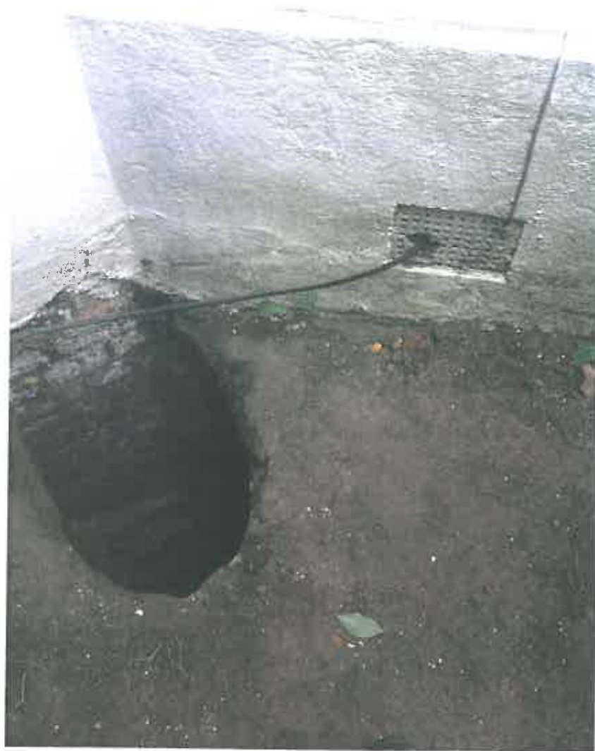
Photo 12 – View of trial pit at front of property. Note the dark edge indicating how the loose fill above foundation level tended to 'bell' out as the hole was excavated.
