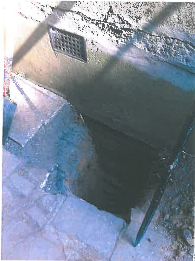
Photo 7 – Trial pit along side access passage
