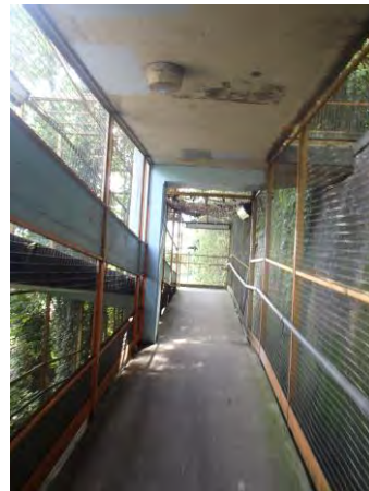
d) Ramps to Mill Lane
