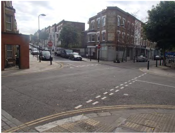
a) Messina Ave / Kingsgate Road raised junction table
