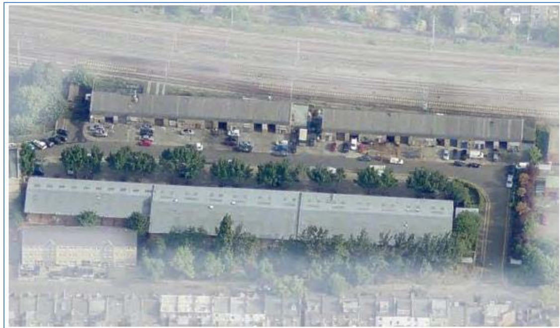
Reproduced from the Kingsgate Primary School and Liddell Road Feasibility Study, Penoyre & Prasad, 2013
