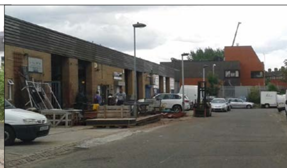
Looking towards the northeast: steel fixing and garage businesses
