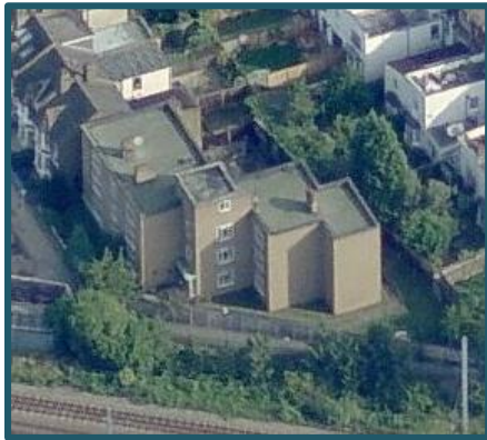
A three storey residential block located to the north west of the development site.
